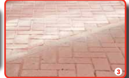
After approximately 1 hour, the surface is set, excess sand is brushed off and the area can be opened to traffic
