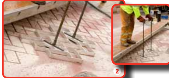
Sand is broadcast over the material to stop the stamp tool sticking while the pattern is imprinted
