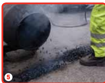
5 Fibrescreed RC100MTR stone/bitumen topping mix is added (if required depending on planed depth)
