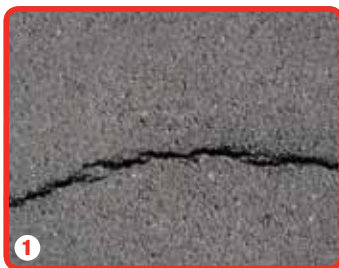
1 Cracks appear in road surface due to heavy trafficking, adverse weather conditions, etc
