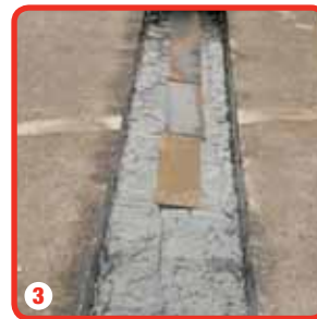
3 Embedding steel plates
