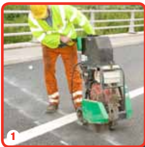
1 Cutting the recess
