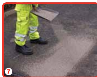
7 Aggregate is broadcast over the surface to provide an appropriate skid resistance level
