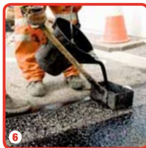
6 Applying finishing layer
