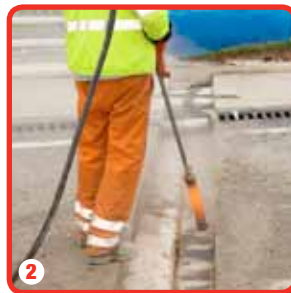
2 Preparing the recess
