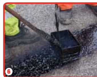
6 Filled crack is screeded over with Fibrescreed RC100MTR bitumen to create a watertight seal
