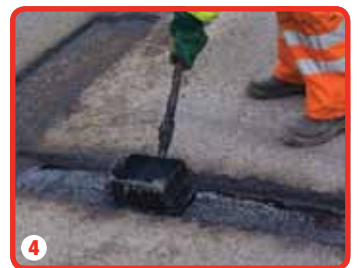
4 Base of recess is sealed with Fibrescreed RC100MTR bitumen
